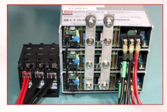
Connect the wires as shown above, matching the wires on the terminal block with the BIC-2200 AC/N, AC/L, and ground connections. The terminal block features three line connections supporting up to 2/0 AWG to an electrical panel.
